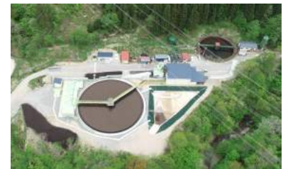
Acid mine drainage treatment facilities (Yatani Mine)
