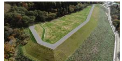
Reinforcement work by soil stabilization at the Yatani Mine Tailings Dam (completion)
