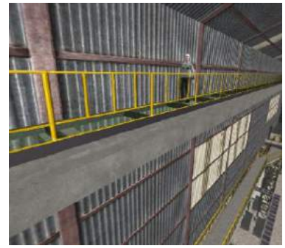
Falling accidents (stepping through the floor)
