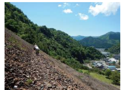
Tailings dam management (Ikuno Mine)
