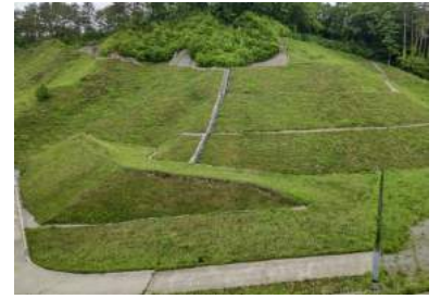
Contamination containment work (Komagi Mine)
