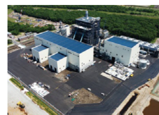
The Yufutsu Energy Center currently under construction
