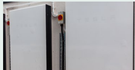
40kW of battery storage
