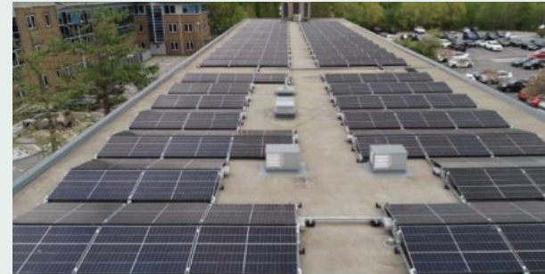
100kW of PV generating 80MWh of electricity per year.
