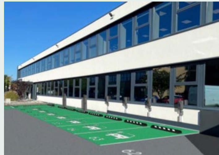
8x22kW Etrac EV sockets
